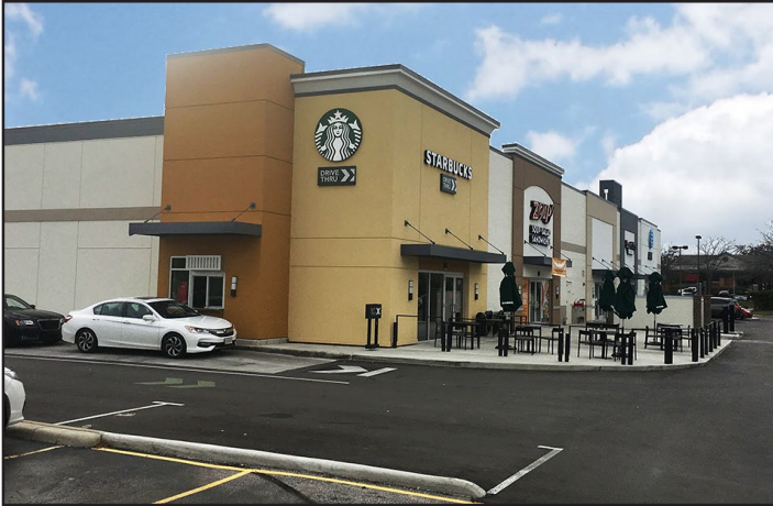
View facing Southwest
