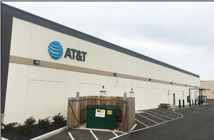
View facing North - AT&T side of building
