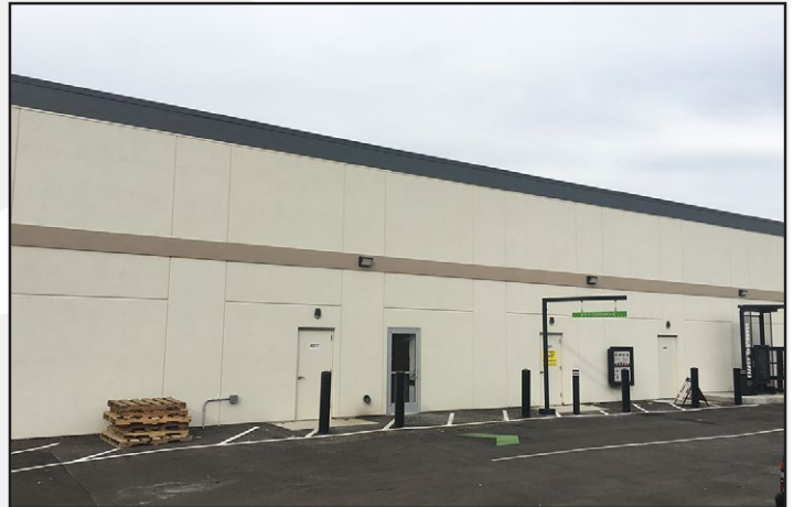
View facing North - Starbucks side of building
